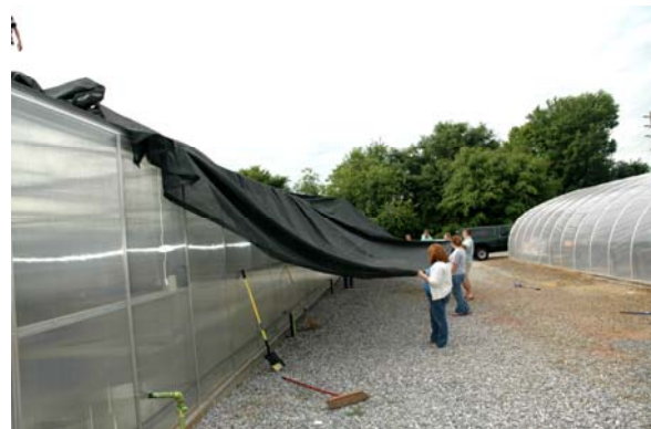
Teachers learning how to apply shade cloth without crawling up on the greenhouse roof.
